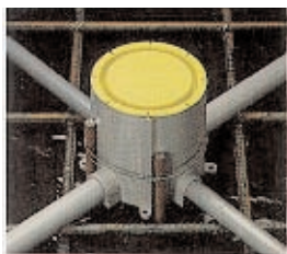
Step 1: Set box using tie-down stakes for on-grade installations or fasten to concrete form for above-grade installations complying with local building codes/regulations.
