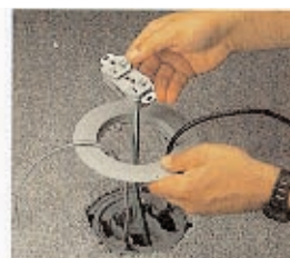
Step 4: To permit future retrofits, mechanically fasten adapter ring using mounting hardware provided, or permanently fasten with glue.
