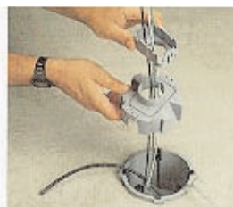
Step 3: Cut and install PFBT1 low-voltage divider as per instructions. Pull wires: receptacle wires go through tube, voice and data cables run outside of tube.
