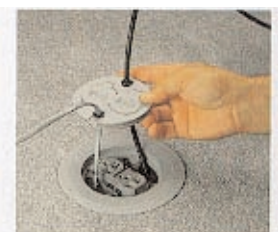
Step 5: Fasten receptacle into carpet flange recess. Feed voice/data cables through punched-out openings on plastic floor box cover. Fasten cover to receptacle.
